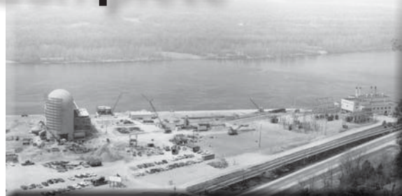
LACBWR construction on the Genoa Site; reactor building under construction. Both photos circa 1967.
